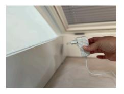
Battery-powered motor – drill 2 holes in the cuff for the AKU battery holder, 10 cm and 33 cm from the upstand corner, maximum 5 cm from the top edge of the upstand. Screw the holder with the screws provided, connect the supply cable to the battery and insert the battery into the holder. Note: The socket for the power cable is also used to connect the charger.
