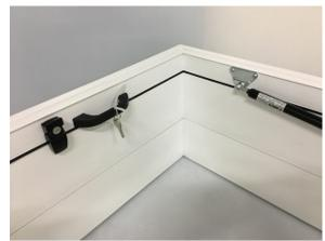
It is always necessary to close and secure skydome during rain, wind and snow, to prevent any damage to hinges and openers.
